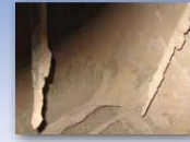
No More Build-Up
